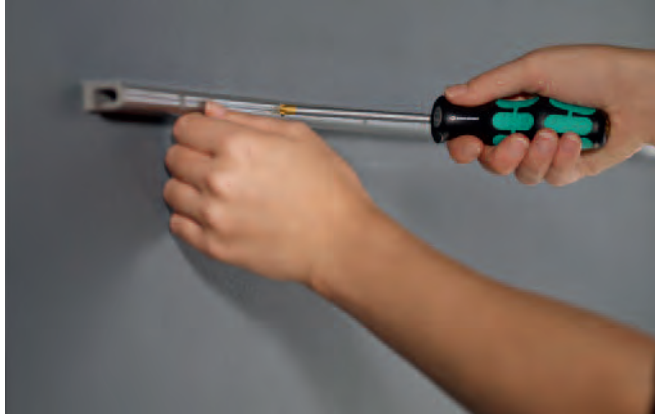
Screw the plastic profile to the wall ...
